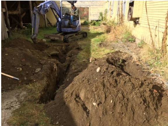
Photograph 3. Area of test pit excavation.
