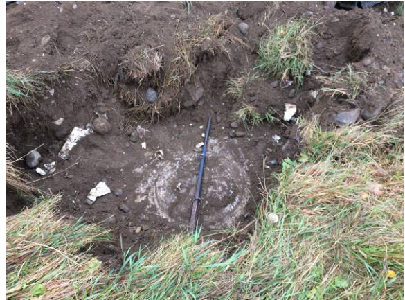
Photograph 4. Top of former septic tank.
